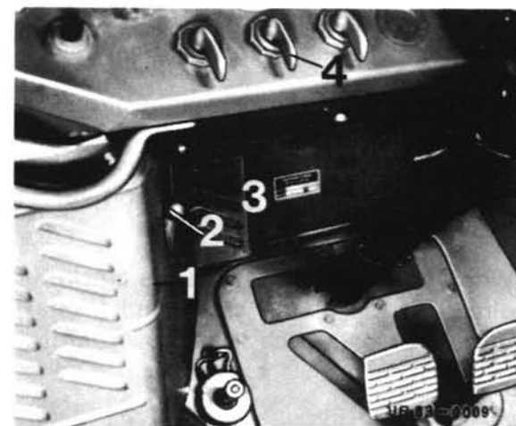
Figure 25 Heating and ventilation system 404.1
